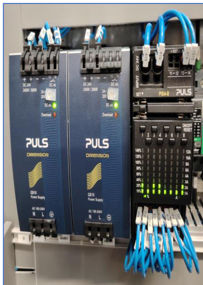
(Figure 3 - Dual Power Supplies)
