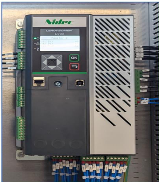
(Figure 1 - Nidec D700 Excitation Controller)
